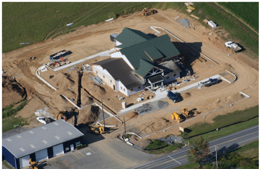
Photo 1: Aerial Photo of Tilden Under Construction
